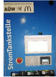
Figure 4: Public multi system fast charging station Source: B.A.U.M. Consult
