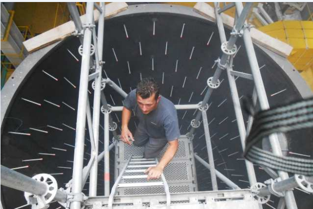
Gasifier inside view during construction
